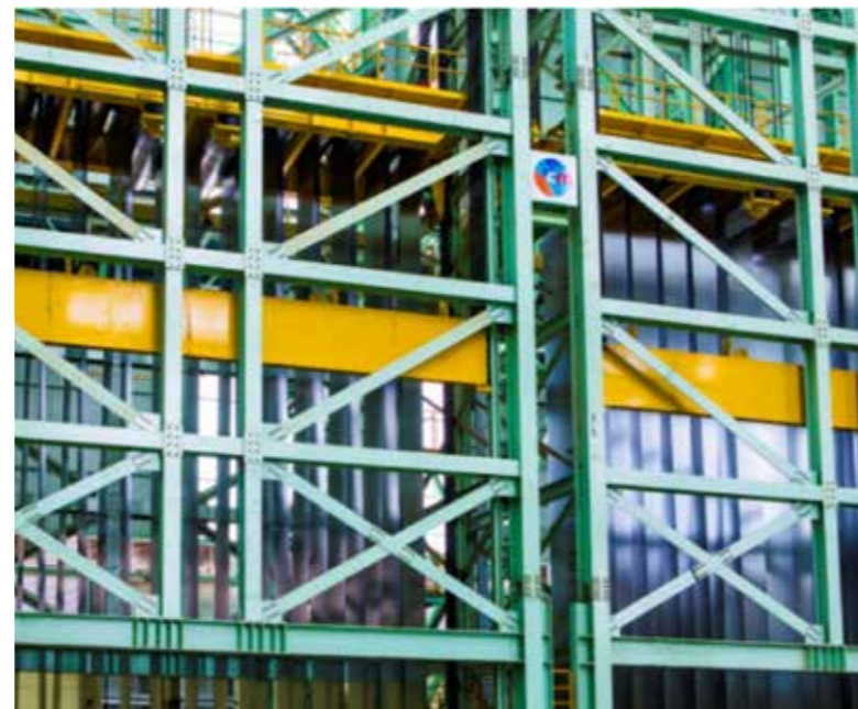
▲ Double accumulator on Combi CAL-CGL, for automotive quality strip, VAMA, China
