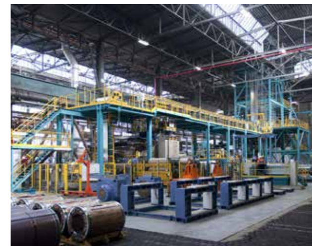
▲ Complete in-line skin pass mill and post treatment section for automotive applications at ArcelorMittal Eisenhüttenstadt
